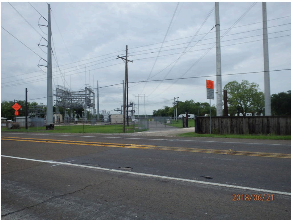
18. Northeast adjoining electrical sub-station across Fannett Road
