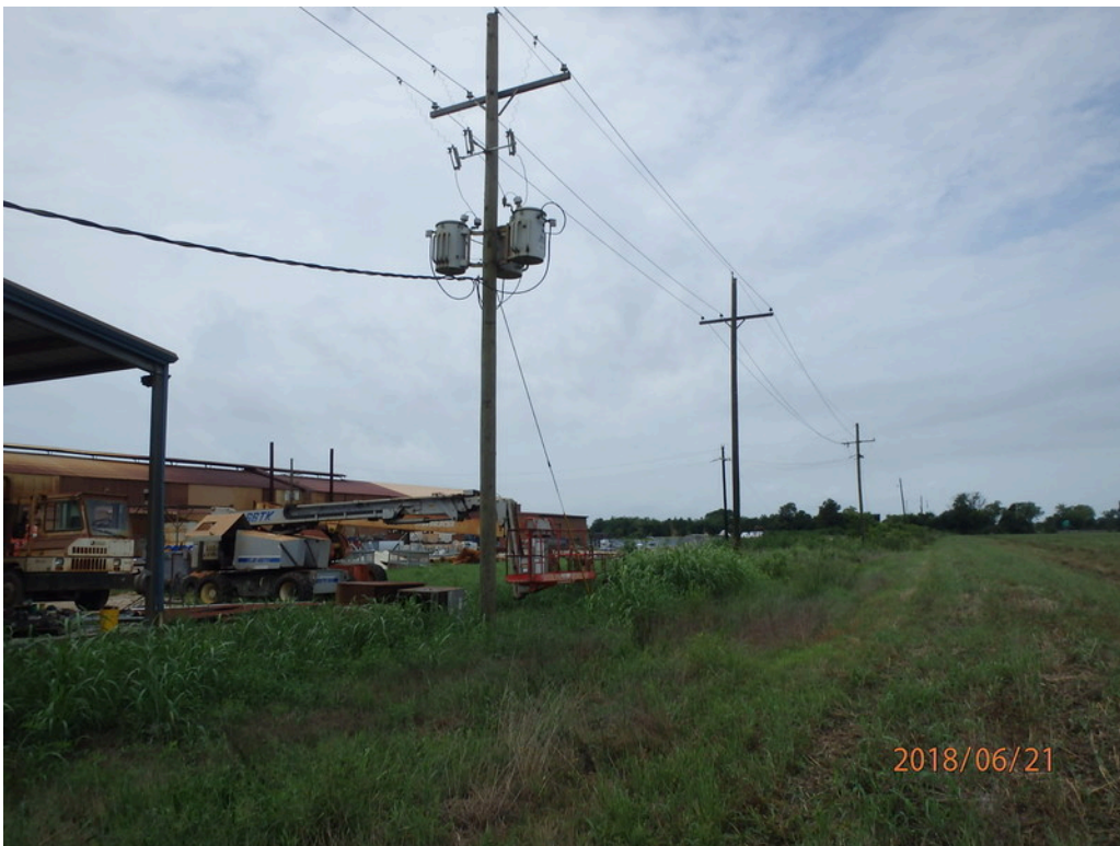
34. View of AZZ Galvanizing property to the south
