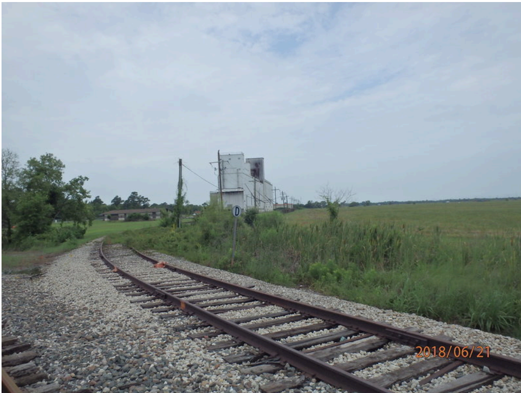
27. View west along south property boundary
