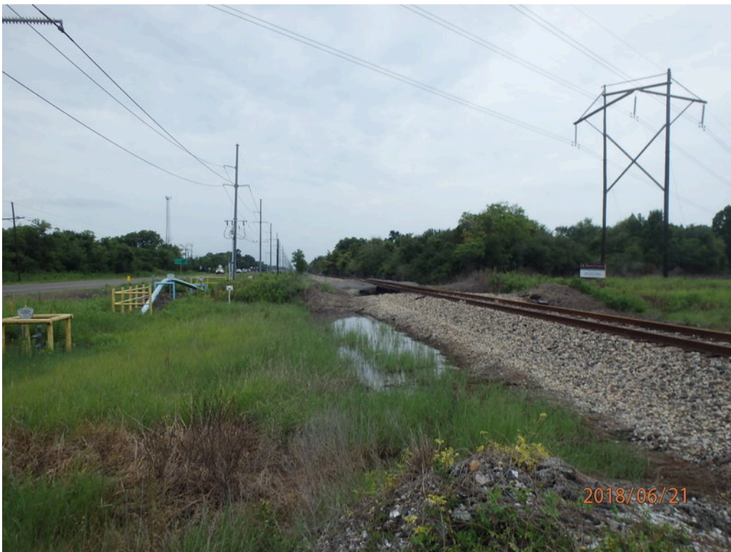
20. Railroad tracks located along southeast property boundary
