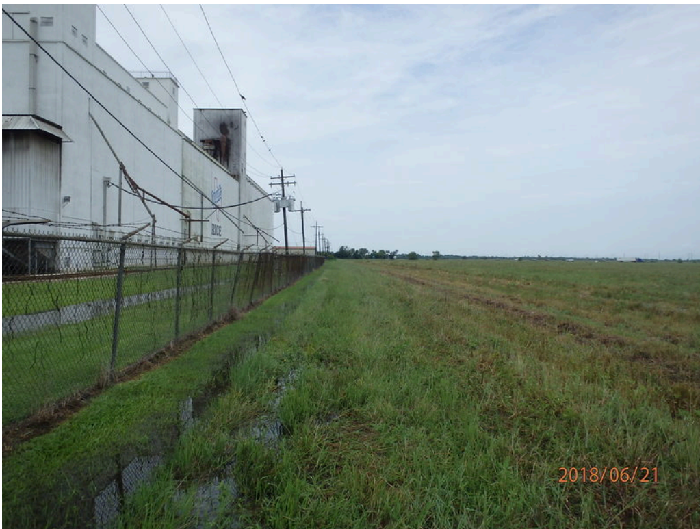
30. Continued view west along southwest property boundary
