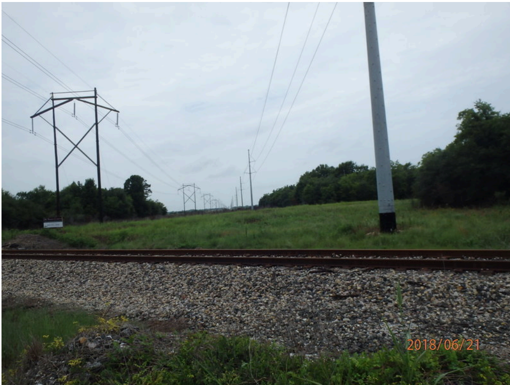
19. View west along onsite overhead electrical easement from Fannett Road
