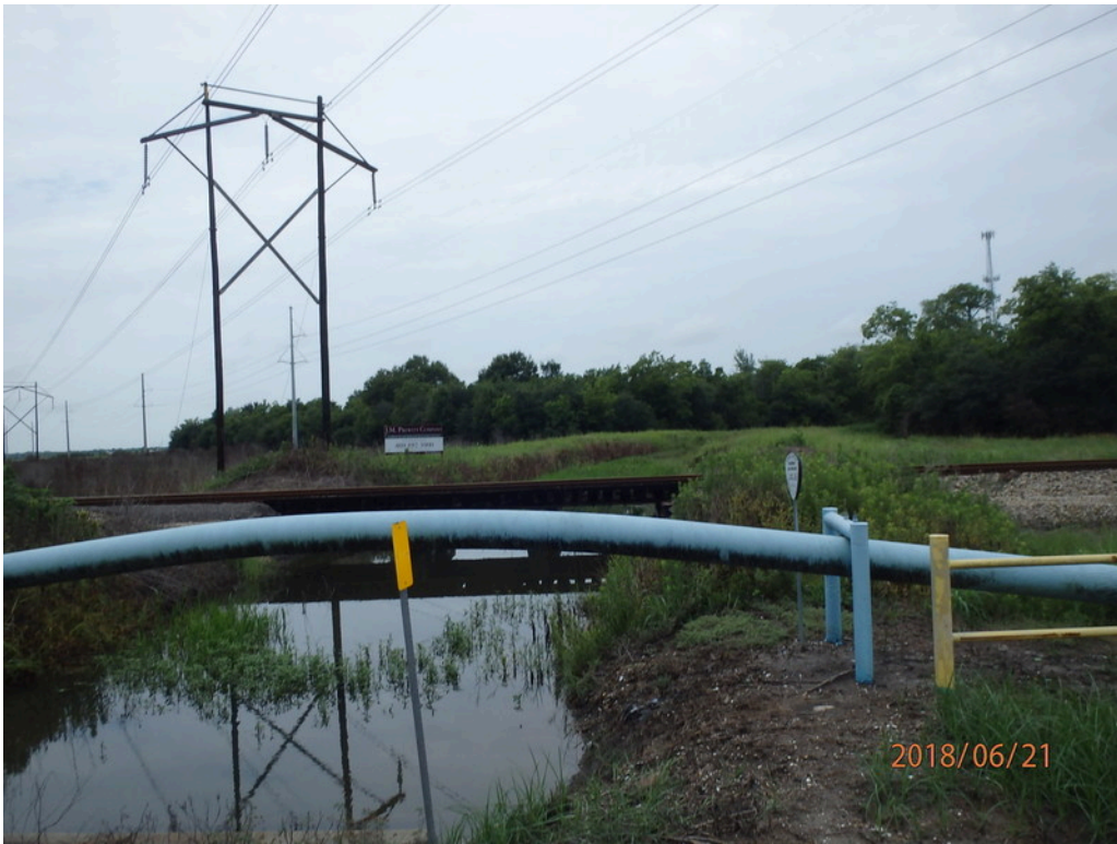
21. Pipeline along southeast property boundary
