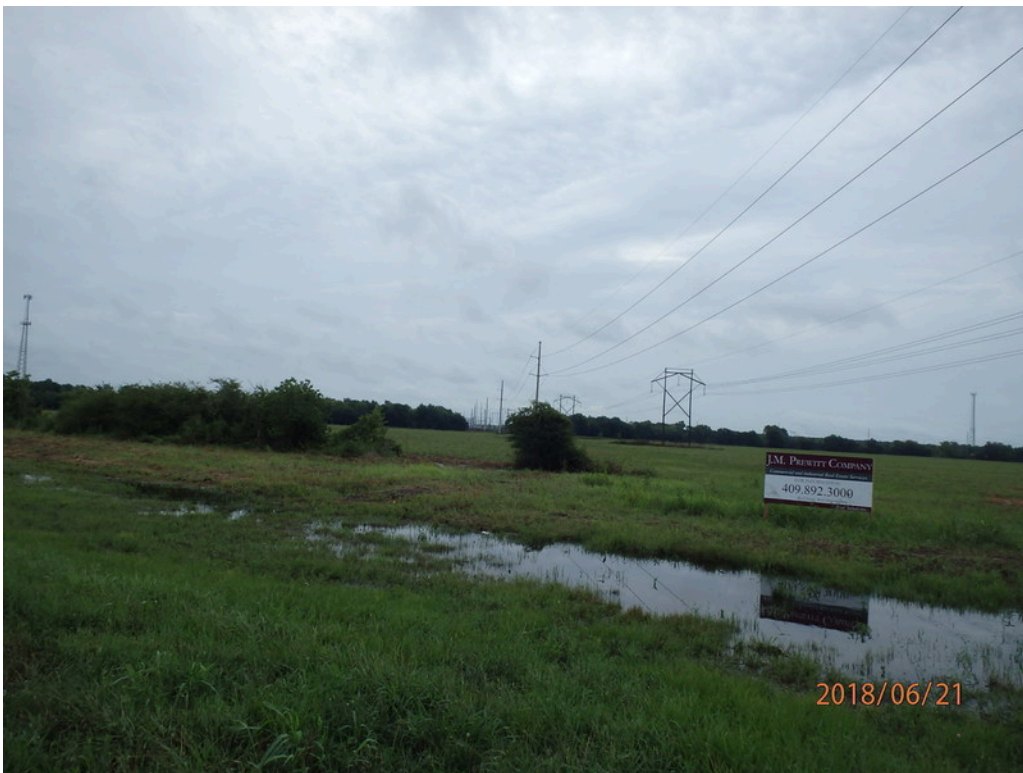
8. View southeast along onsite overhead electrical easement from IH-10
